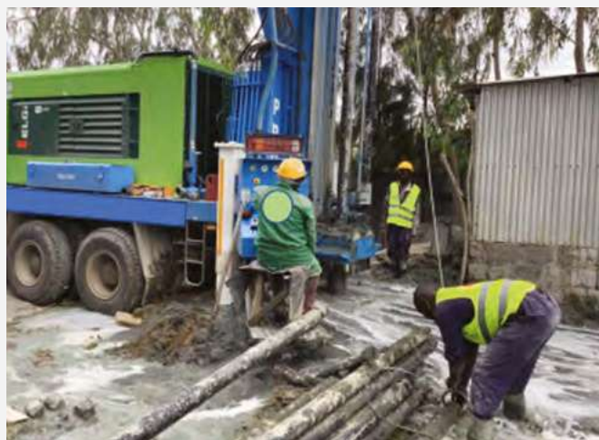
Drilling of bore hole
